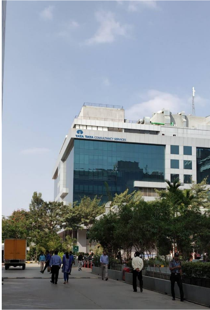
Figure 14 TCS Building, Bengaluru
