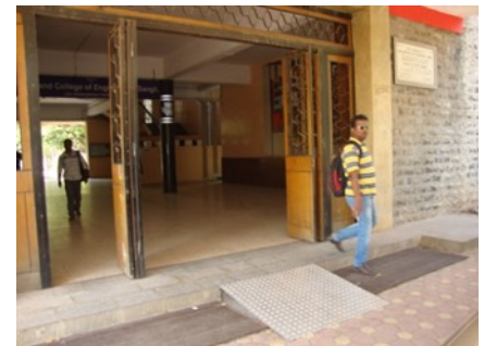
Ramp in Main Building Entrance
