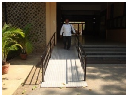
Ramp in Main Building
