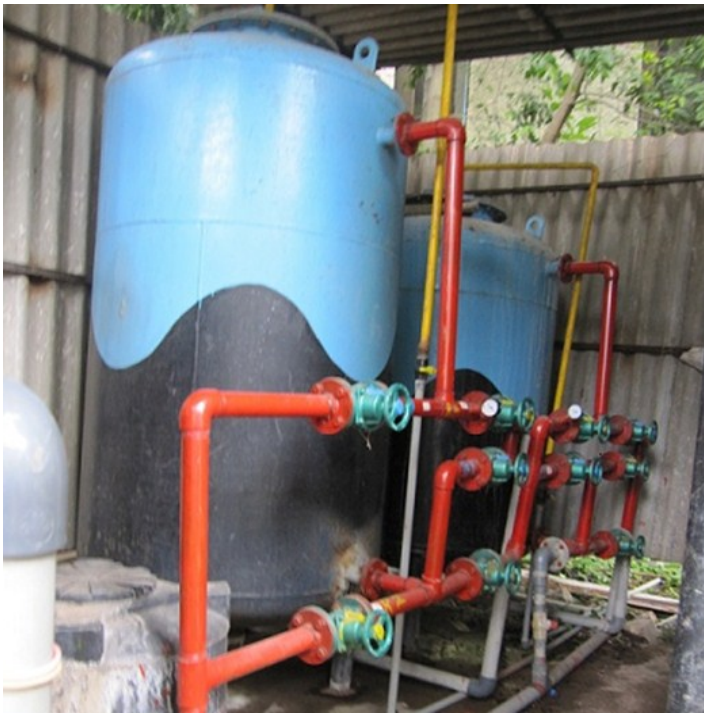
Water Filtration Plant of 50000 liters capacity and Distribution System Power Substation with 325 KVA sanctioned Capacity and Generator set of 125 kVA capacity along with PLC and SCADA system caters to the electricity needs during load shedding.
