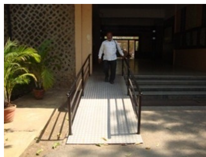
Ramp in Main Building
