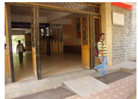
Ramp in Main Building Entrance
