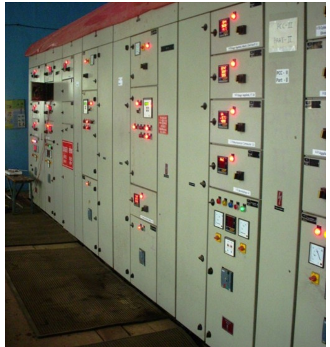
Water Filtration Plant of 50000 liters capacity and Distribution System Power Substation with 325 KVA sanctioned Capacity and Generator set of 125 kVA capacity along with PLC and SCADA system caters to the electricity needs during load shedding.
