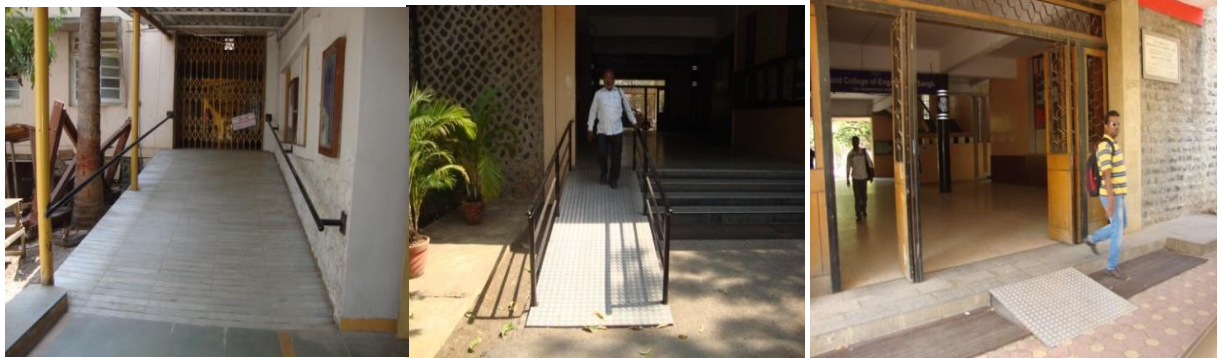
Ramp in Quadrangle-Civil Dept Ramp in Main Building Ramp in Main Building Entrance
